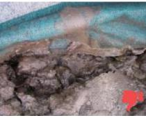
Not buried deep enough & ground poorly compacted.
